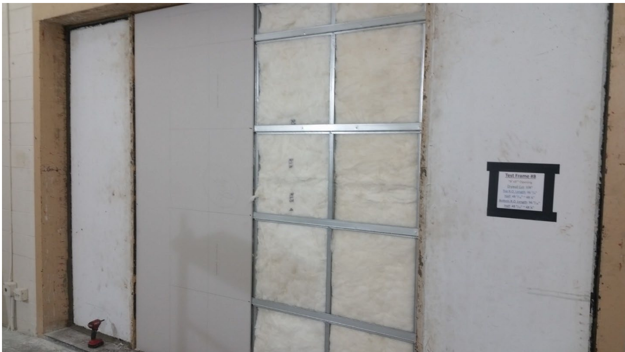
Figure 6 – Source room side base layer gypsum partially installed
