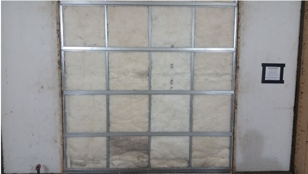
Figure 5 – Insulation installed in stud cavities, viewed from source room side
