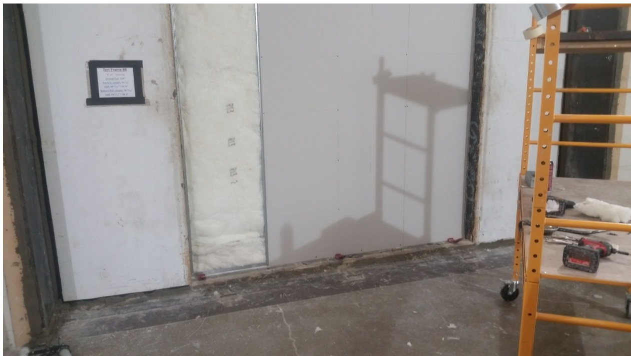
Figure 8 – Receive room side gypsum partially installed, view from receive room
