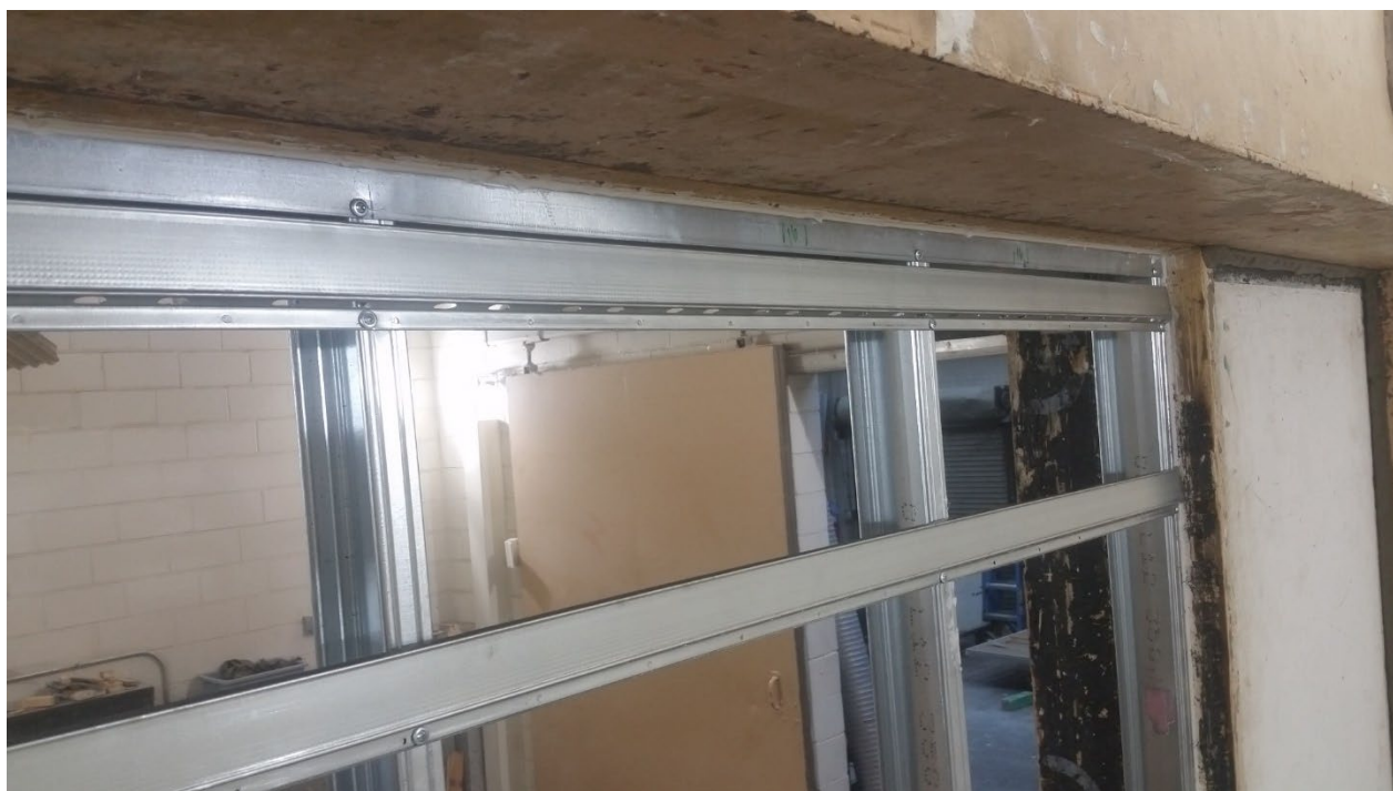
Figure 4 – Detail of studs fastened to track and resilient channel fastened to studs
