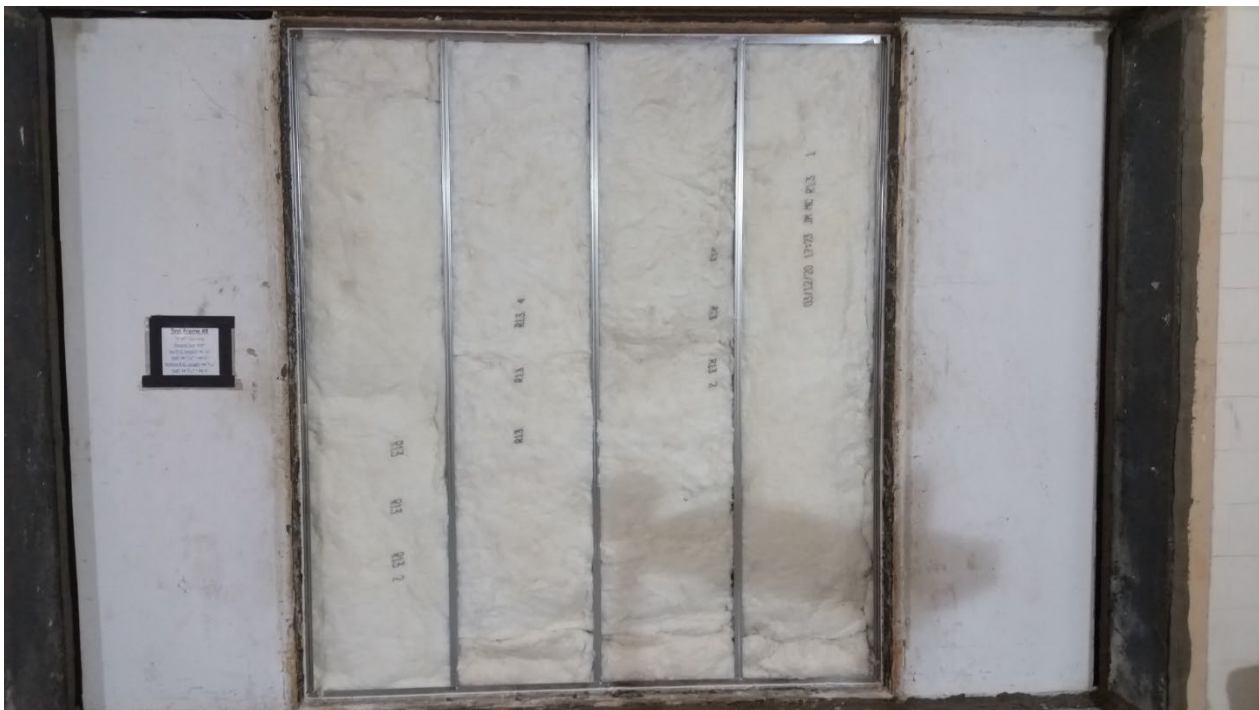
Figure 8 – Insulation installed in stud cavities, viewed from receive room side
