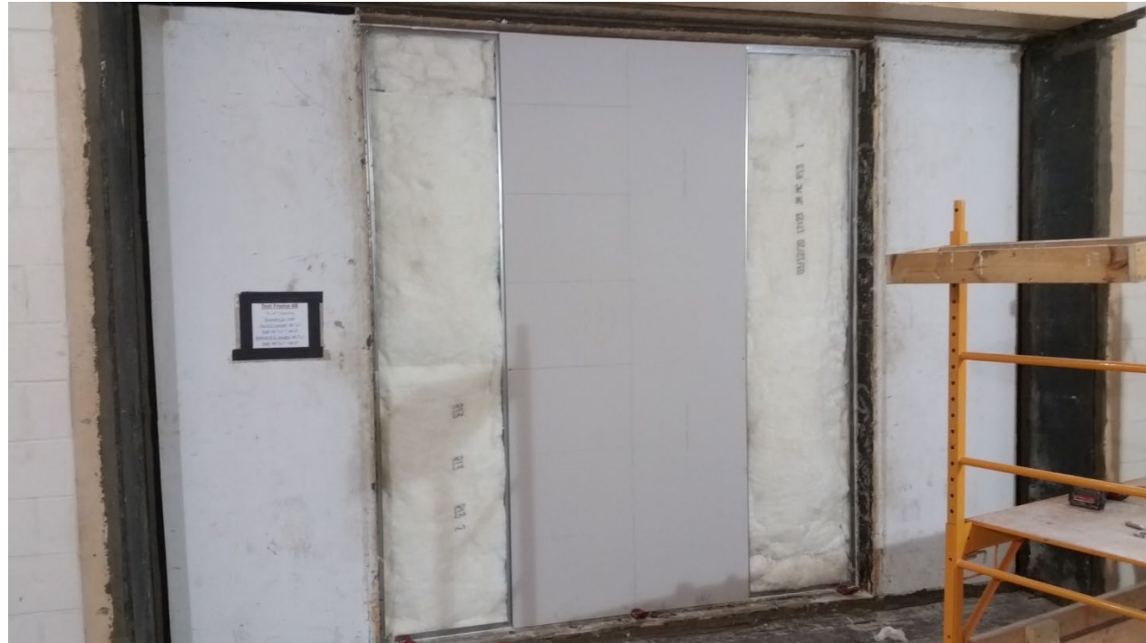
Figure 9 – Gypsum board partially installed on receive room side of studs
