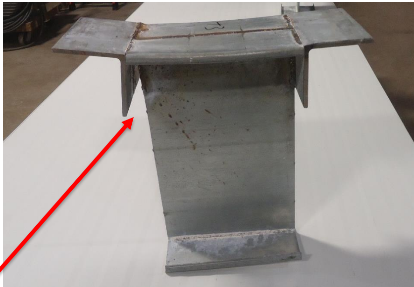
VERT. WELD BROKE AT ANGLE TO JOIST WEB CONNECTION
